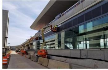
Hanging Framework for Cladding Panel Installation South Side of Escalators at Dulles Station
