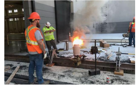
Thermite Welding Replacement Insulated Joint 'Plug' in Place
