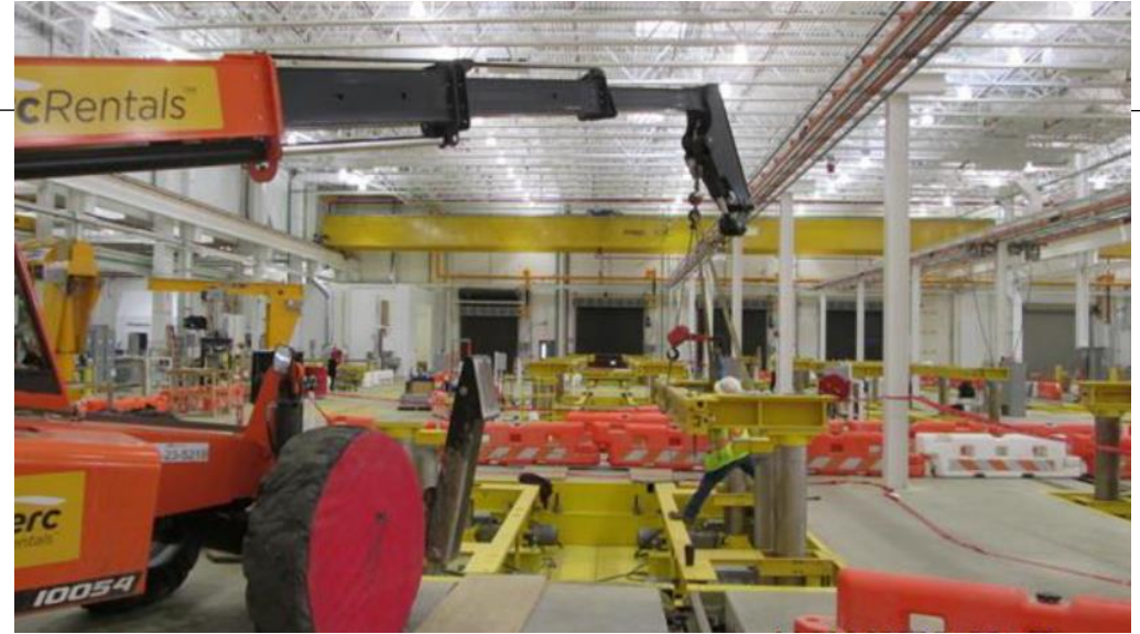
Hoist Installation in Service and Inspection Building (SIB)
