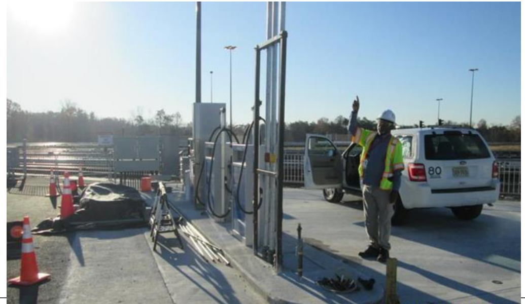
Inspecting Fuel Dispensing Point
