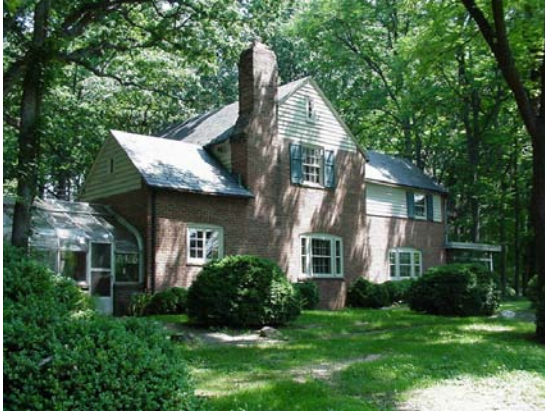
Figure 3, White residence. Source: FCPA, 2002.
