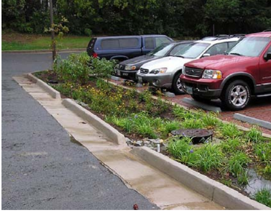
Figure 29, bioswales at Providence RECenter, Falls Church, Virginia. Source: FCPA, 2005.
