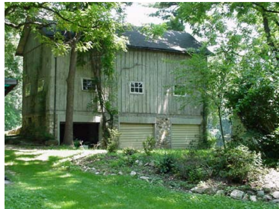
Figure 10, barn. Source: FCPA, 2002.
