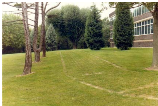
Figure 28, fire access lane paved with Grasscrete® pavers. Source: Courtesy of Grass Concrete Limited, 2005.
