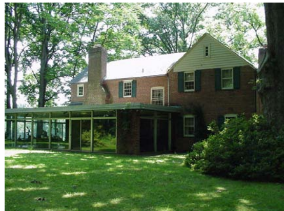
Figure 31, White residence, glass porch at back. Source: FCPA, 2005.
