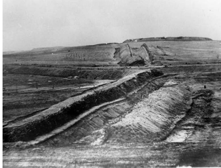
Figure 7: Civil War Earthworks in Centreville
