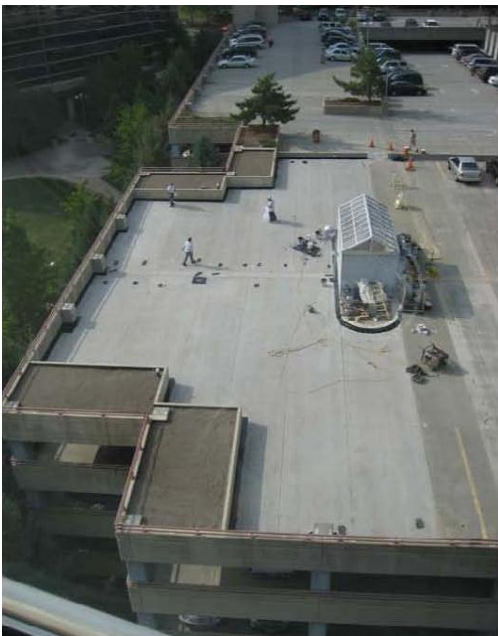
Photo 4.8 Before Green Roof
