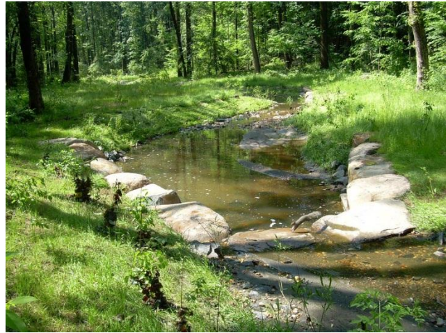
Photo 4.12 Rock Vane in Completed Stream Restoration in Reston, Virginia Source: Reston Association
