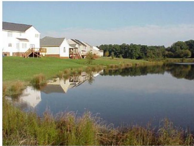
Photo 4.3 Retention Basin Source: Virginia Stormwater Management Handbook
