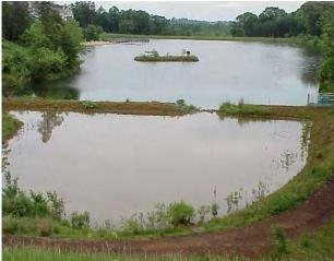
Figure 4-2: Wet stormwater pond with forebay
