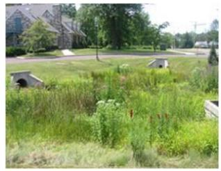
Figure 4-1: Dry stormwater pond
