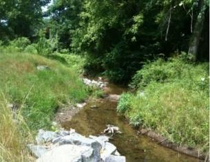
Figure 4-7: Cross vane added to stream
