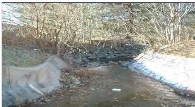
Concrete lined portion of Dead Run
