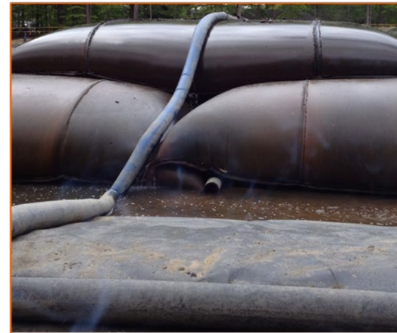
Step 3: Sediment Dewatering
