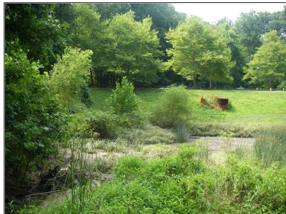
Figure 4-3: Engineered stormwater wetland (Source: Fairfax County)
