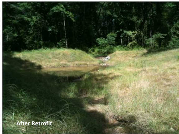
Figure 4-18: Outfall improvement (Source: Fairfax County)
