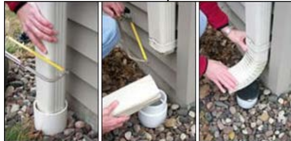
Figure 4-21: Disconnecting a downspout (Source: City of Toronto)
