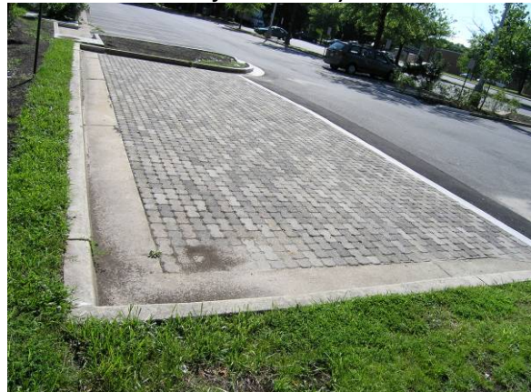
Figure 4-22: Permeable pavement blocks in a parking lot (Source: Fairfax County)
