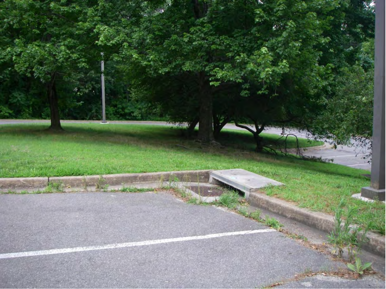
BE9509_1.jpg: View of Parking lot inlet
