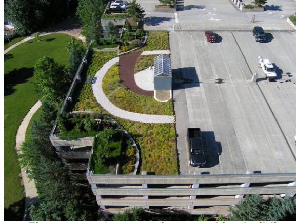
Figure 4-11: Green roof on a parking building (Source: Fairfax County)
