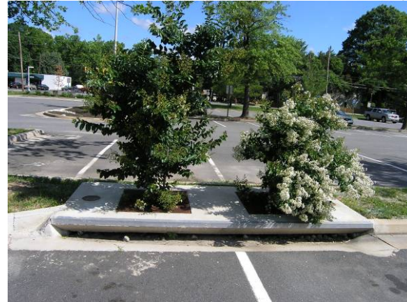
Figure 4-10: Tree box filter (Source: Fairfax County)
