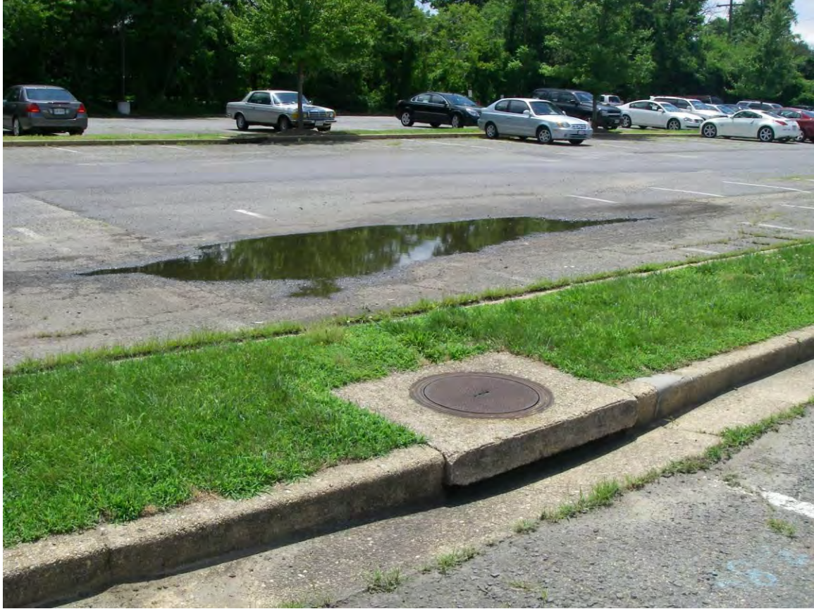
BE9504_1.jpg: View of existing inlet and median in parking lot
