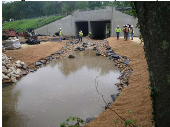
Figure 4-17: New replacement culvert (Source: KCI)
