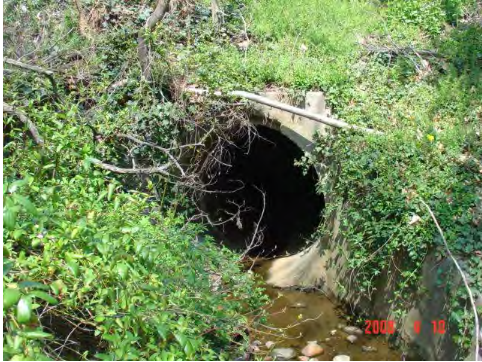
BE9600_1.jpg: Upstream side of culvert on Yale Drive
