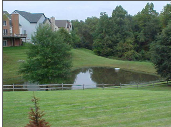
Figure 4-2: Stormwater Management wet pond (Source: Fairfax County)
