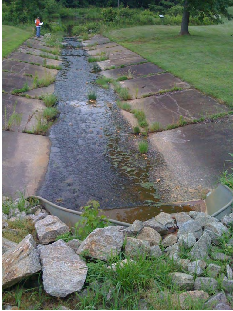
DC9213_1.jpg: Concrete channel at Greendale Golf Course
