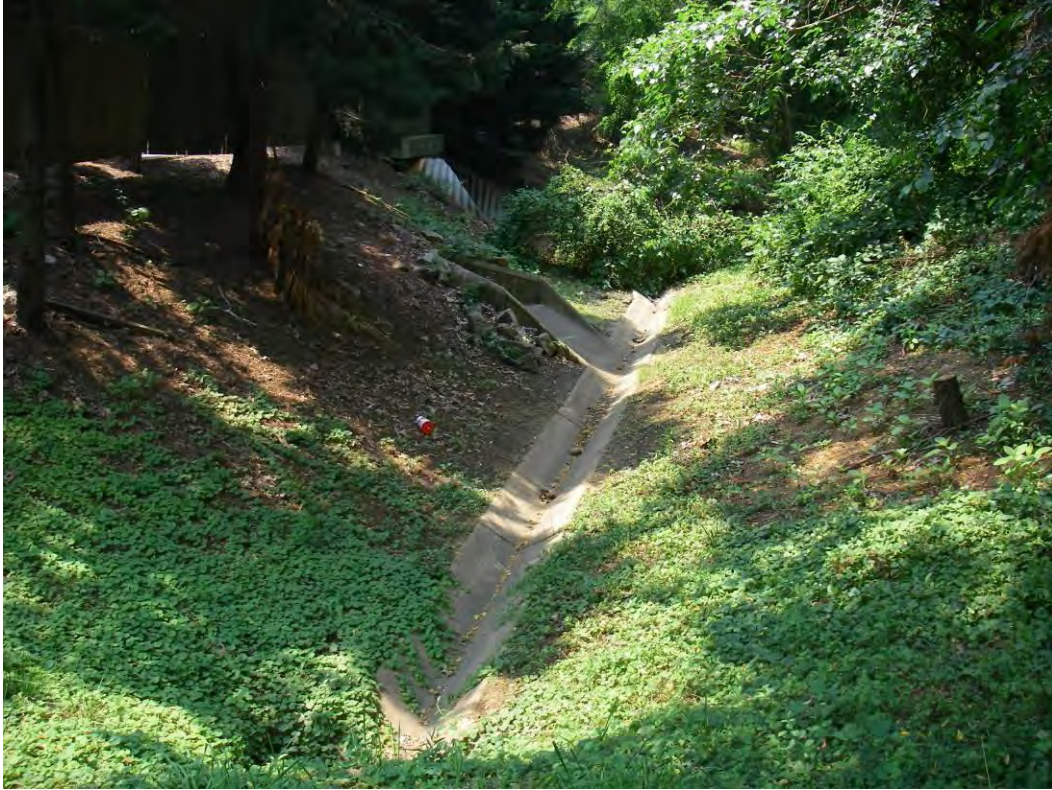
FM9104_1.jpg: View of inflow to pond
