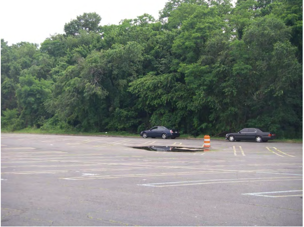
BE9501_1.jpg: View of existing parking lot
