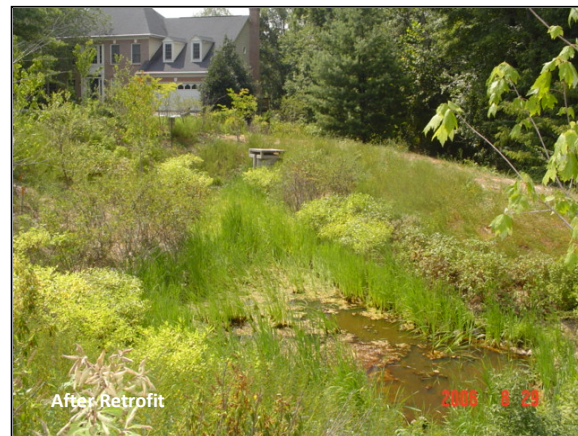
Figure 4-4: Stormwater dry pond retrofit (Source: Fairfax County)
