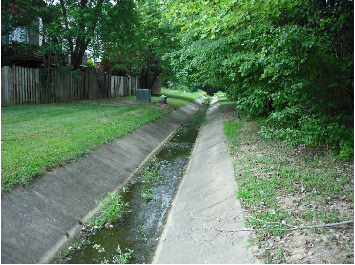
DC9210_1.jpg: View of the existing concrete channel
