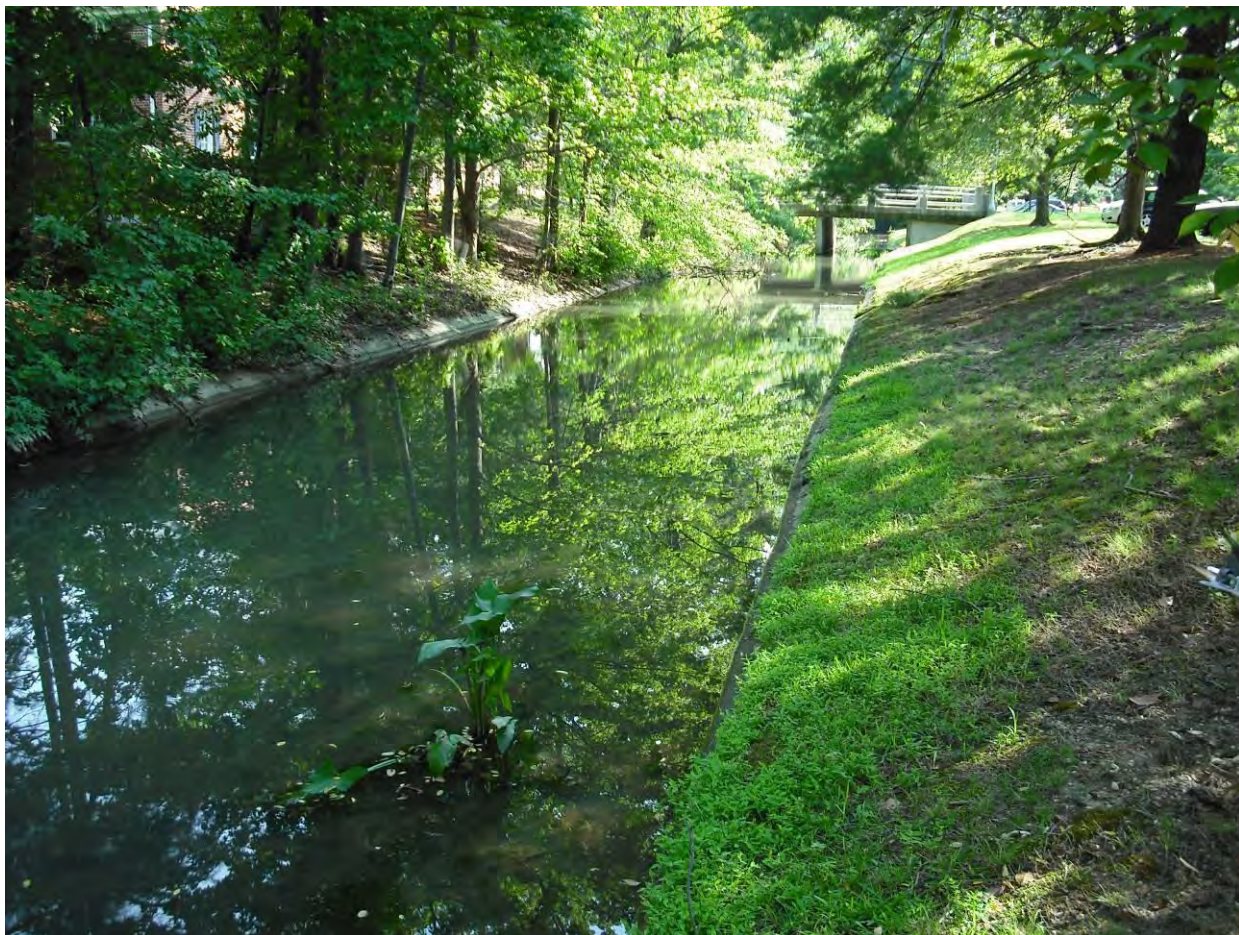
BE9201_1.jpg: View of concrete channel section
