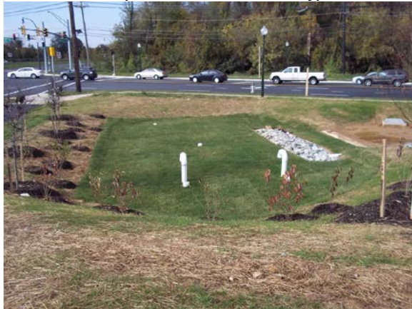
Figure 4-12: Sand filter along MD355 (Source: KCI)
