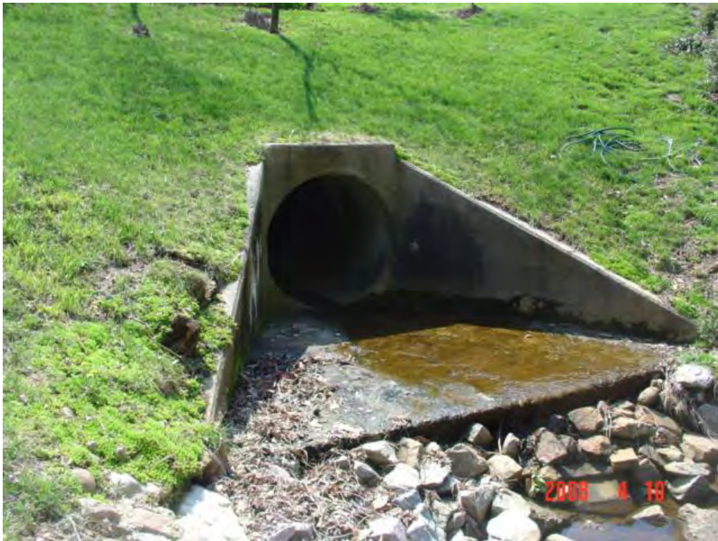
BE9600_2.jpg: Downstream side of culvert on Yale Drive
