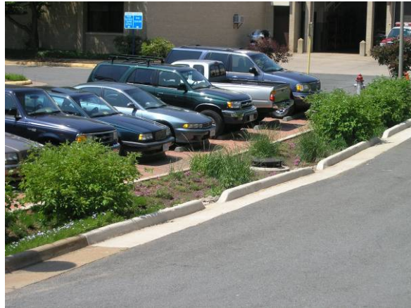
Figure 4-8: Parking lot bioretention (Source: Fairfax County)
