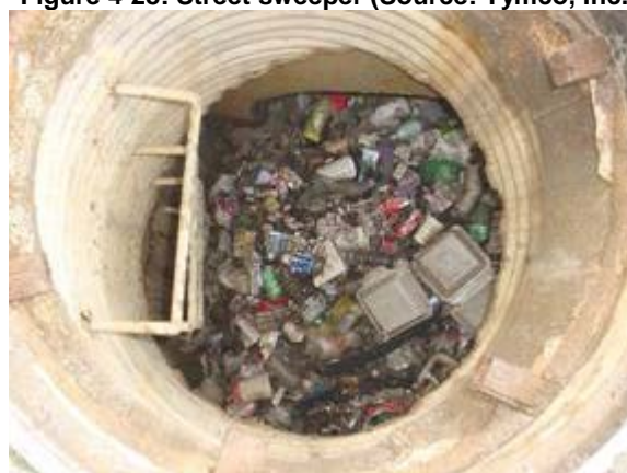
Figure 4-29: Catch basin (Source: Fairfax County)
