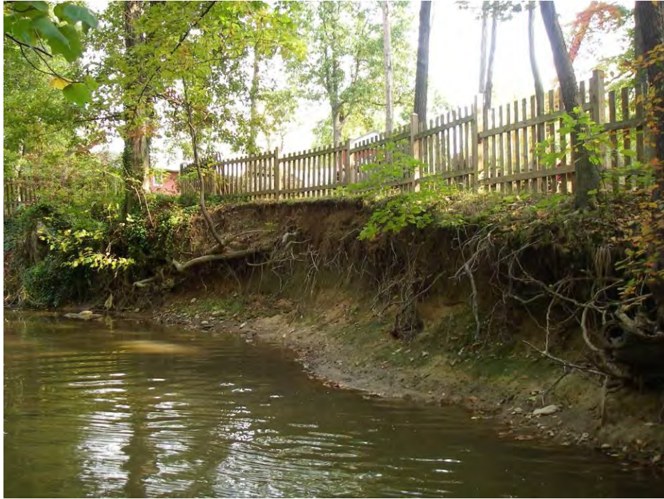
DC9217_1.jpg: Eroded stream banks
