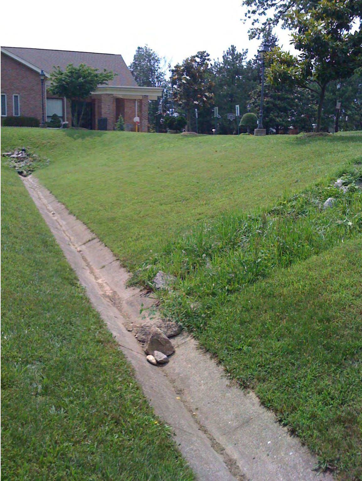
DC9523_1.jpg: View of proposed bioretention site
