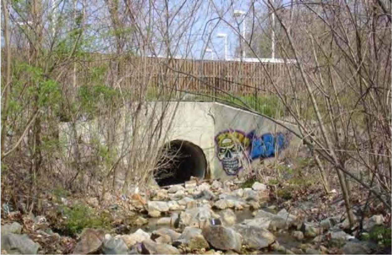
BE9601_1.jpg: View of Pipe downstream of Quander Road
