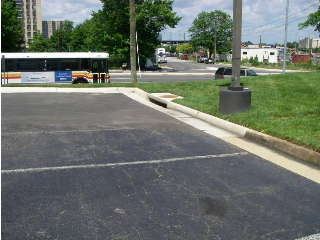
BE9500_1.jpg: View of existing storm drain inlet
