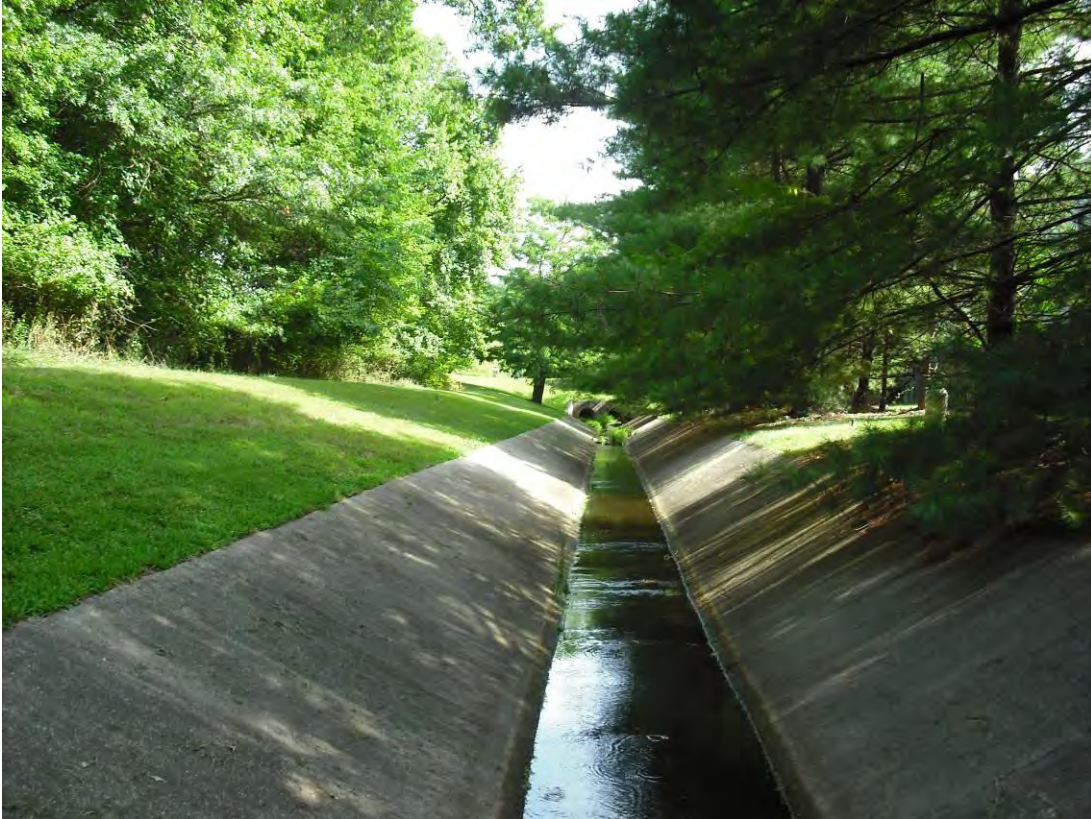
DC9211_1.jpg: View of the existing concrete channel
