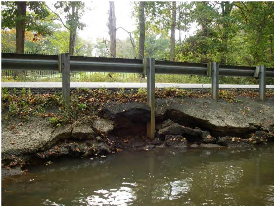
DC9217_2.jpg: Area to be stabilized along Old Mill Road
