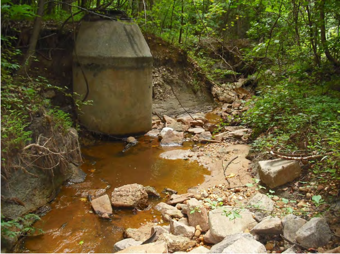
DC9215_1.jpg: View of stream section
