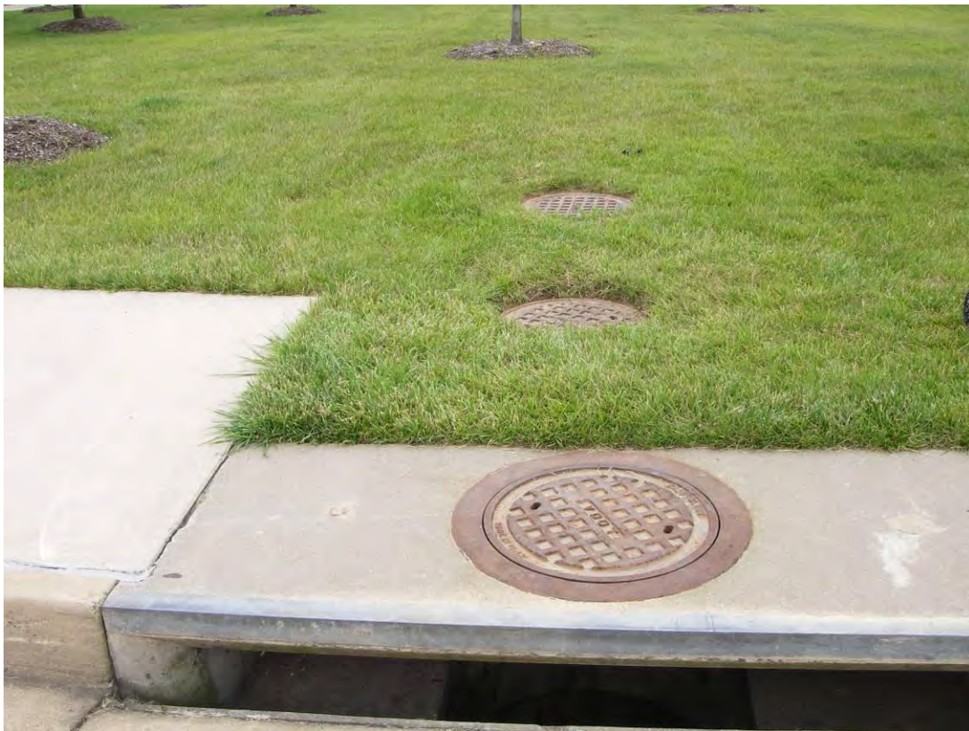
DC9518_2.jpg: Existing inlet in parking lot
