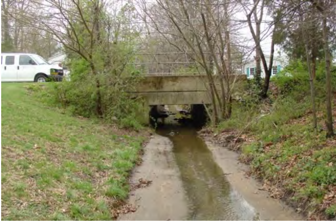
DC9600_1.jpg: View of existing culvert under Ashboro Dr
