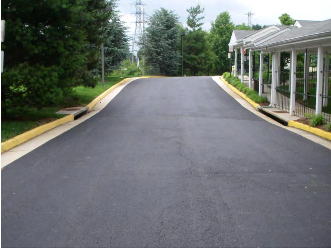
DC9507_1.jpg: View of existing inlets at end of Wescott Hills Way
