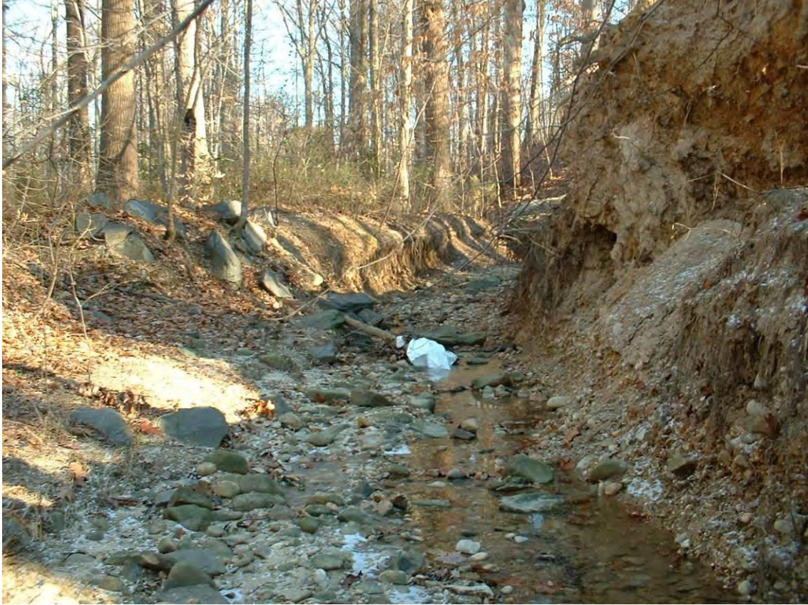
DC9203_1.jpg: View of the eroded stream section
