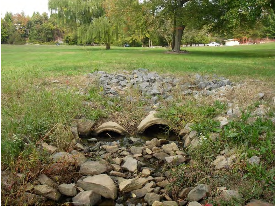
DC9218_1.jpg: Stream to be daylighted
