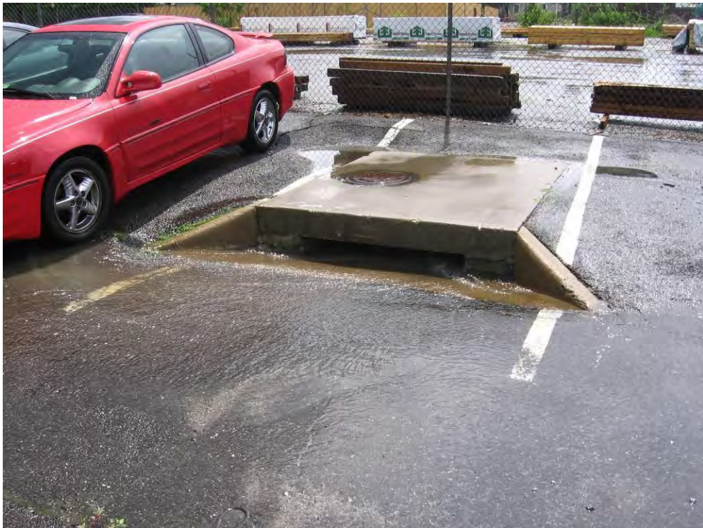
DC9500_2.jpg: View of existing inlet
