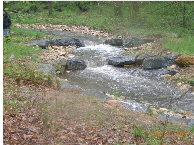
Photo 4.10 Step Pool Channel Source: Arlington County, VA
