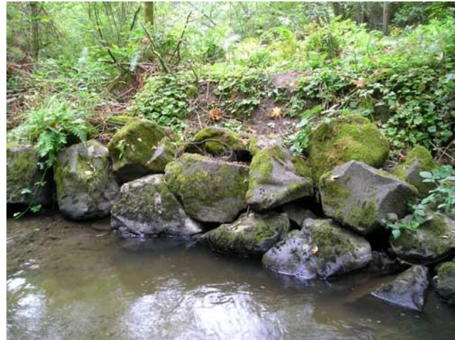
Photo 4.12 Boulder Revetment Source: Center for Watershed Protection
