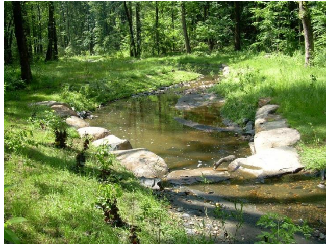
Photo 4.11 Rock Vane in Completed Stream Restoration in Reston, Virginia
