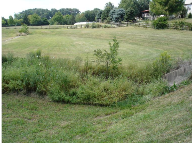
Photo 4.7 Vegetated Water Quality Swale Source: F. X. Browne, Inc.
