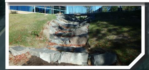
RSC systems (the outfall to the pond) is an open-channel, sand seepage filtering system that utilizes a series of shallow aquatic pools, riffle weir grade controls, native vegetation and underlying sand channel. The system combines features and treatment benefits of swales, infiltration, filtering and wetland practices.
