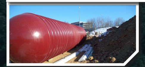
Rainwater is harvested from the top roof and collected in an underground, 25,000-gallon cistern. Water from the cistern is used to irrigate landscaping around the building.
