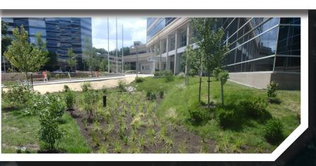
These depressed, landscaped gardens capture and filter During stormwater runoff. storms, runoff temporarily ponds then rapidly filters through a bed of sand, soil, and organic filtering media. Native plants like rushes and sedges help take up and treat stormwater, provide wildlife benefits, and create appealing landscaping.
