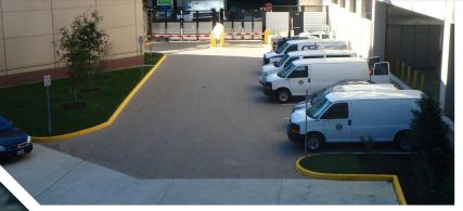
The PSHQ service driveway is paved with permeable pavers. These interlocking brick pavers allow water to drain through the gaps between the bricks into a gravel base below. The water than infiltrates or slow flows into the storm drain system that discharges to the wet pond.
