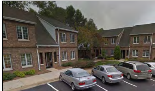
Office units along Bowman Green Drive
