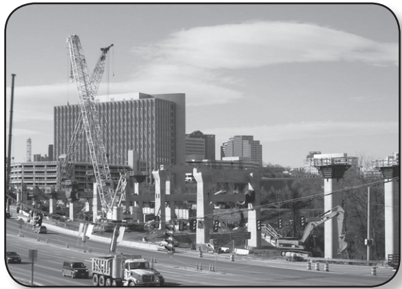
Construction of the Tysons East Station at Route 123 and Coleshire Road (Capital One Headquarters in background).
