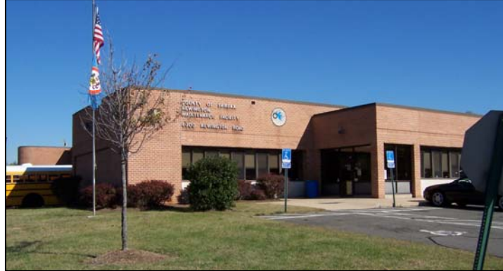
Picture of existing Newington facility
