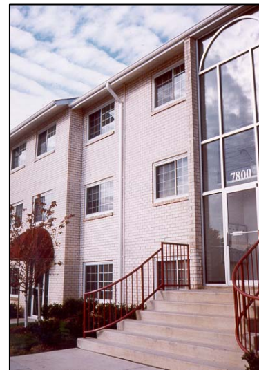
Murraygate Village apartments in Hybla Valley
