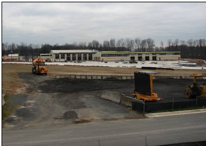
Picture of the West Ox Bus Operations Center under construction, slated for completion in fall 2008.
