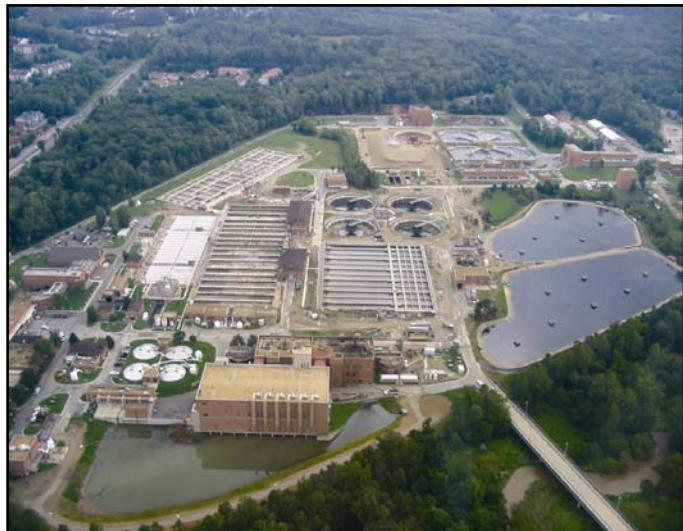
The County's wastewater treatment plant serves an estimated 340,000 households with public sewer service to help maintain a safe and caring community.
