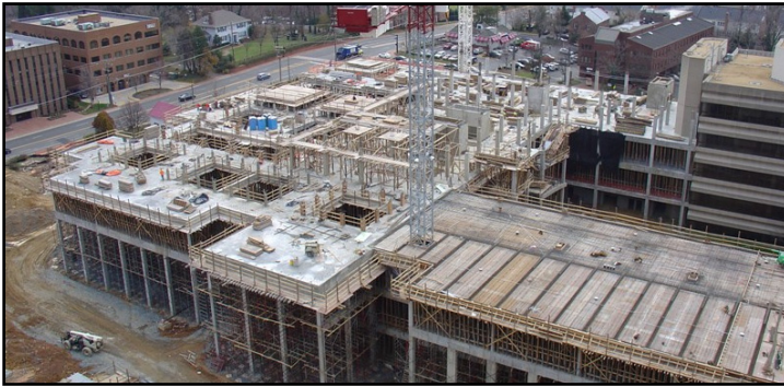
Significant progress is being made on the Courthouse Expansion and Renovation project.
