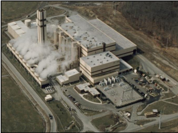
I-95 Energy/Resource Recovery Facility
