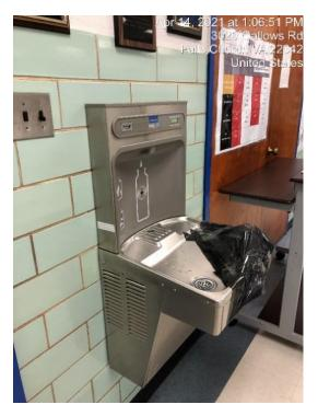
Figure 2-11. Installed Bottle Filling Station at a Current FCPS Middle School (spout currently inoperable due to COVID-19 health and safety regulations).
